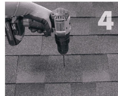
4 If attaching with lag bolt use a 1/4" bit (Lag). Use a 1/8" bit (ST) for attaching with the structural screw. Drill pilot hole into roof and rafter, taking care to drill square to the roof. Do not use mount as a drill guide. Drill a 2" deep hole into rafter.
