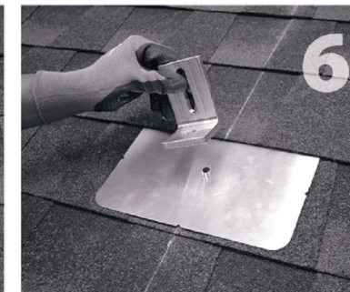
6 Place L-foot onto elevated flute and rotate L-foot to desired orientation.
