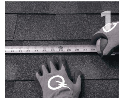
1 Locate, choose, and mark centers of rafters to be mounted. Select the courses of shingles where mounts will be placed.
