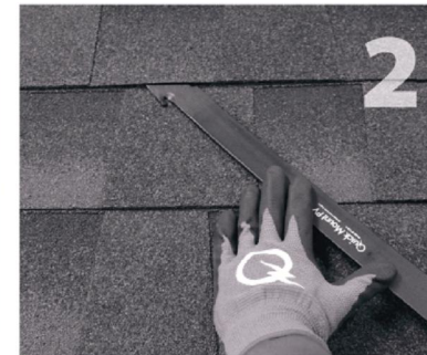
2 Carefully lift composition roof shingle with roofing bar, just above placement of mount. Remove nails as required and backfill holes with approved sealant. See "Proper Flashing Placement" on next page.
