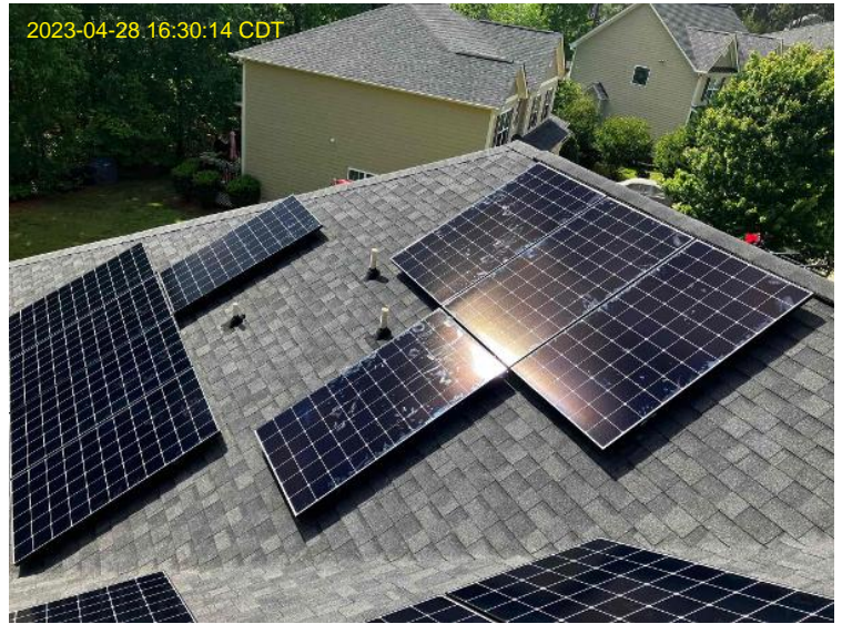
Roof/Array Work / Photo: Overall Array (s)
