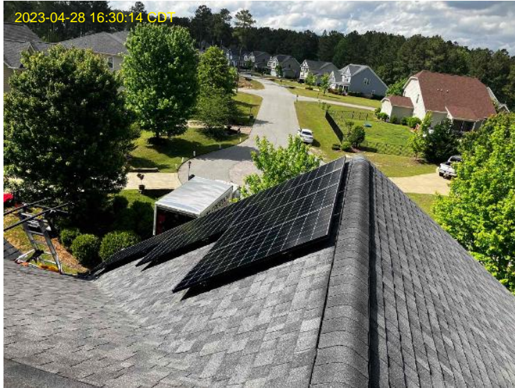
Roof/Array Work / Photo: Overall Array (s)
