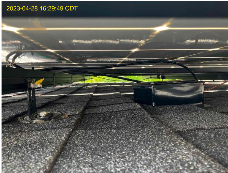
Roof/Array Work / Photo: Under Array (wire management)
