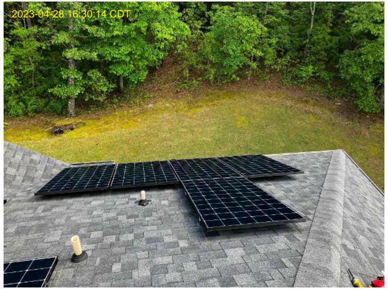
Roof/Array Work / Photo: Overall Array (s)
