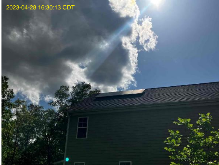
Roof/Array Work / Photo: Overall Array (s)
