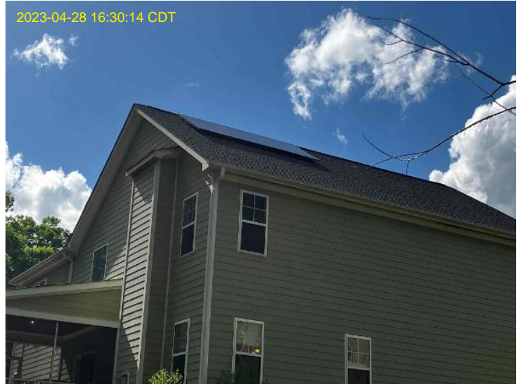
Roof/Array Work / Photo: Overall Array (s)
