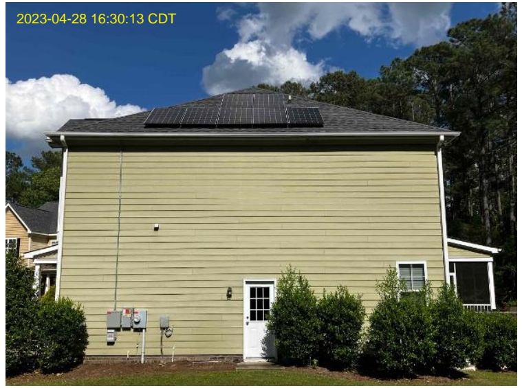
Roof/Array Work / Photo: Overall Array (s)
