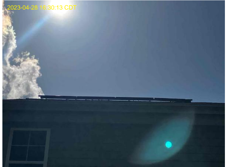
Roof/Array Work / Photo: Overall Array (s)
