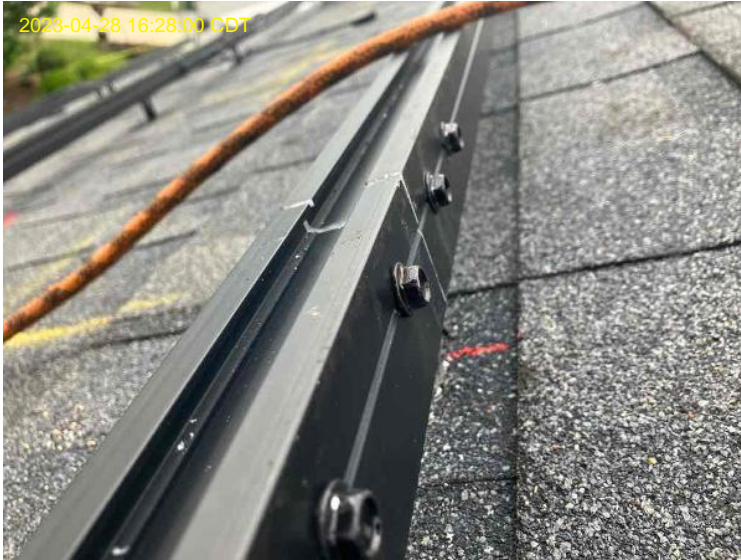
Roof/Array Work / Photo: Flashing/Roof Mount close up (racking)
