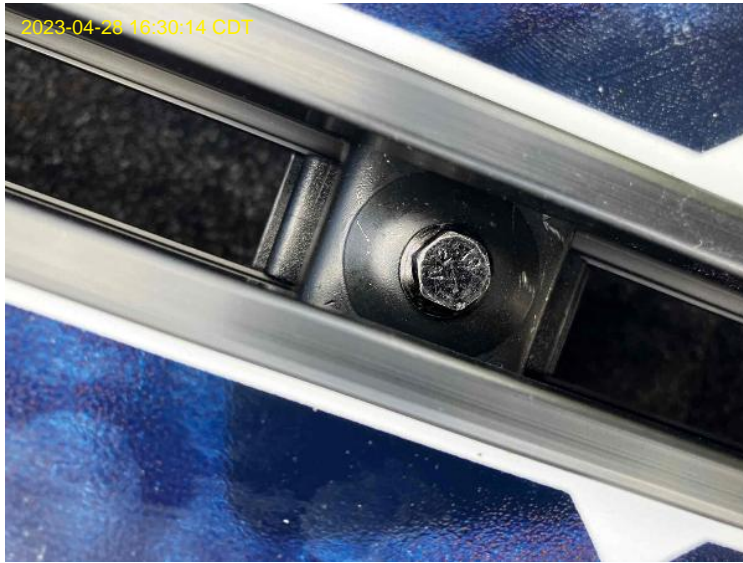
Roof/Array Work / Photo: Overall Array (s)
