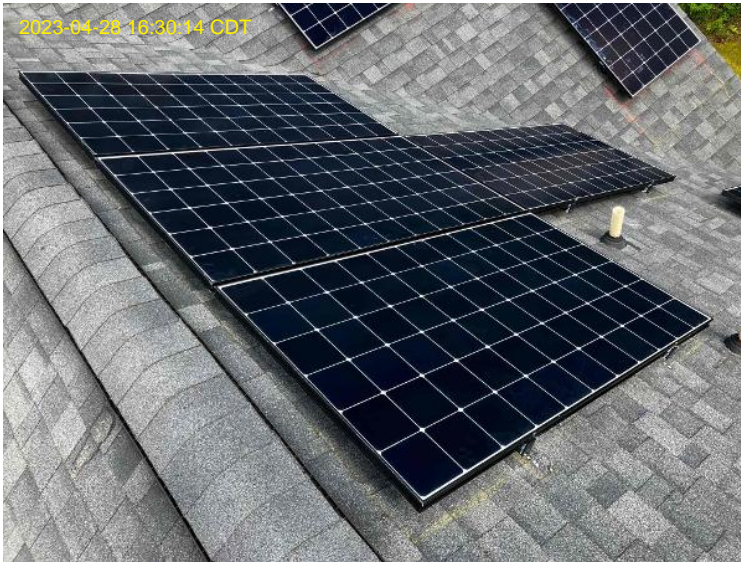
Roof/Array Work / Photo: Overall Array (s)
