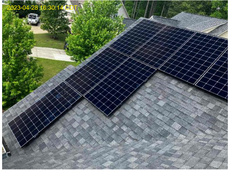
Roof/Array Work / Photo: Overall Array (s)
