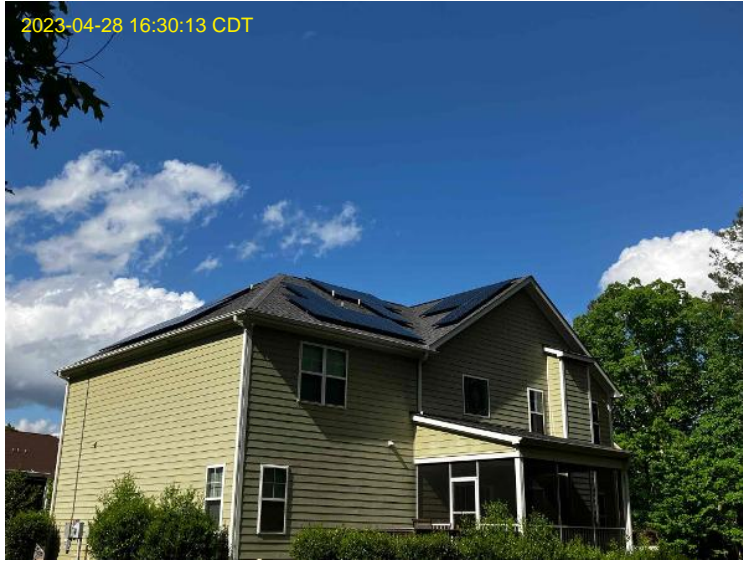
Roof/Array Work / Photo: Overall Array (s)
