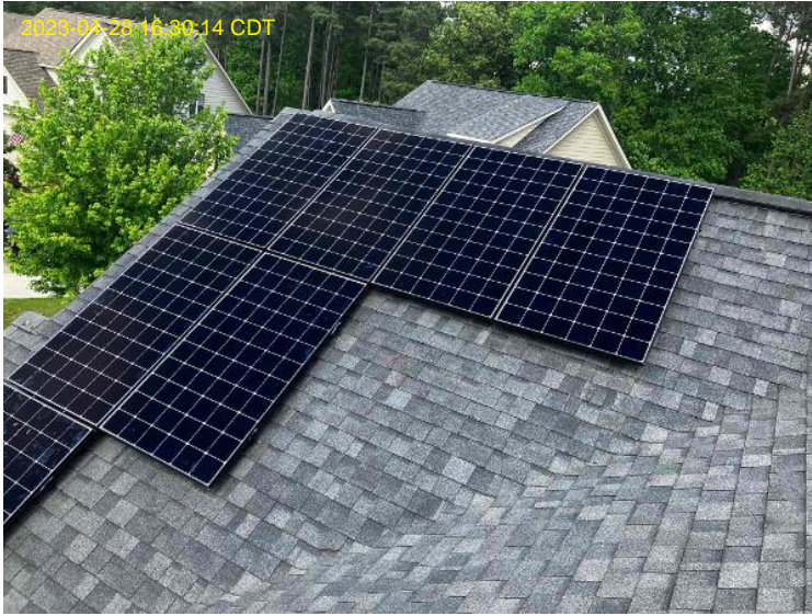
Roof/Array Work / Photo: Overall Array (s)
