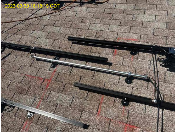
Roof/Array Work / Photo: Conduit Run(s)
