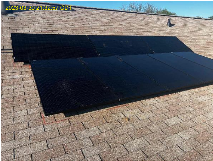
Roof/Array Work / Photo: Overall Array (s)
