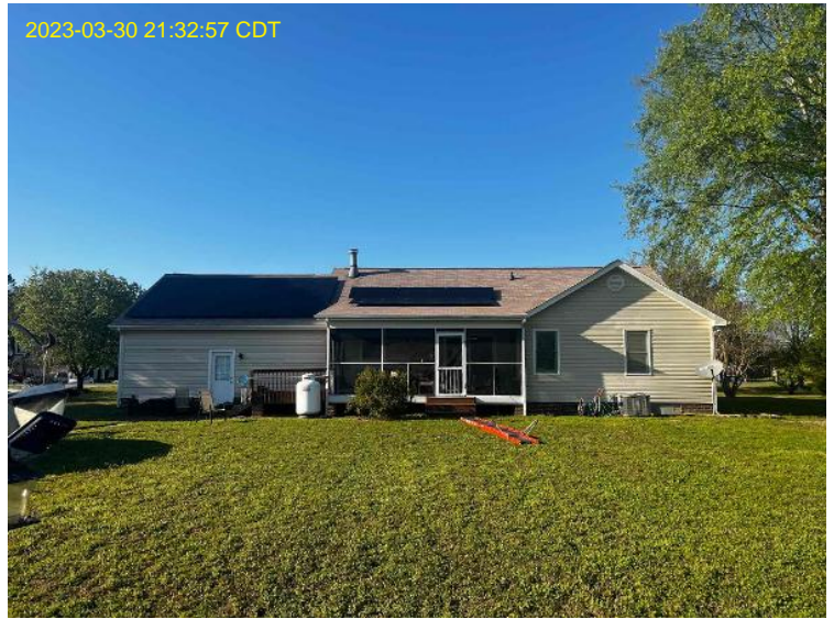
Roof/Array Work / Photo: Overall Array (s)
