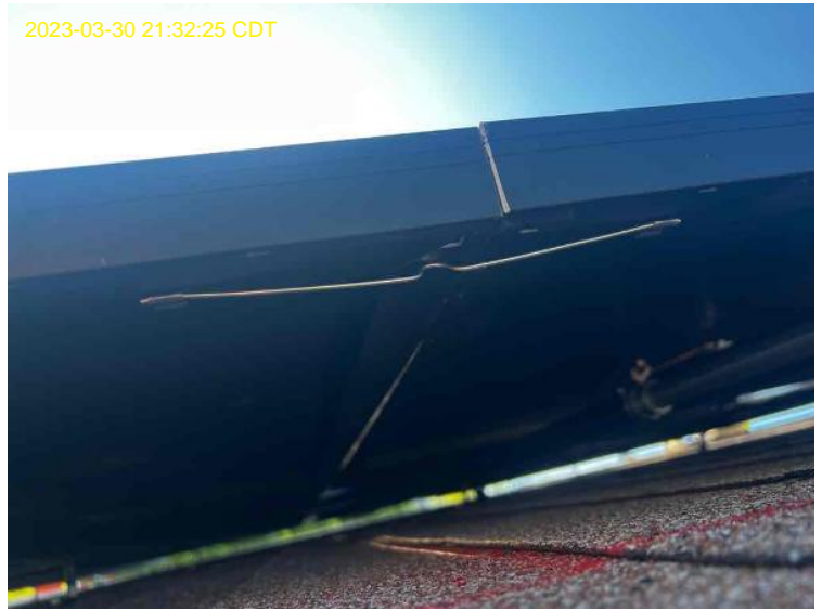
Roof/Array Work / Photo: Array Grounding Jumper(s)
