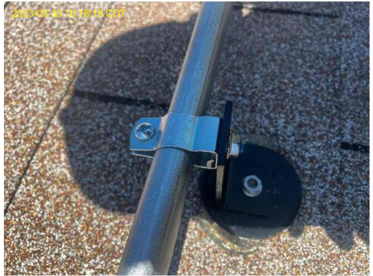
Roof/Array Work / Photo: Conduit Run(s)
