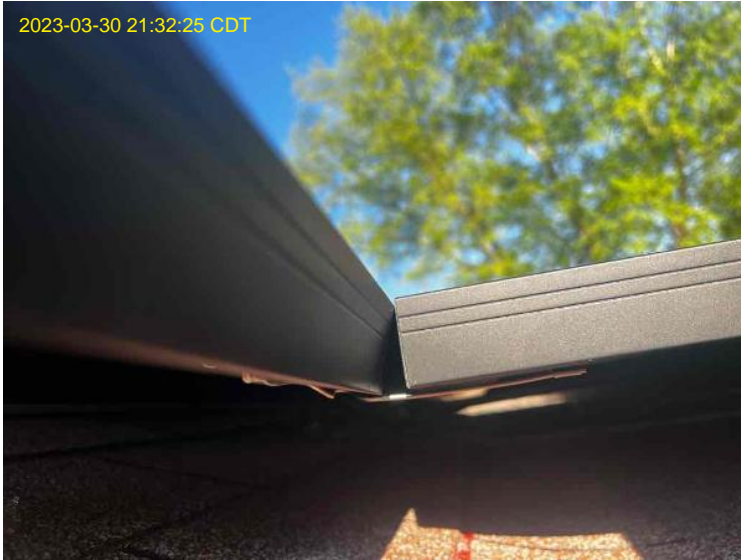
Roof/Array Work / Photo: Array Grounding Jumper(s)
