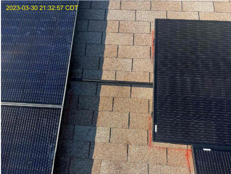
Roof/Array Work / Photo: Overall Array (s)
