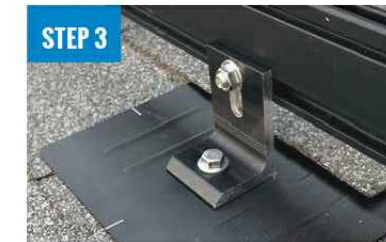
ATTACH L-FOOT TO RAIL
