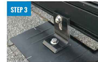
ATTACH L-FOOT TO RAIL
