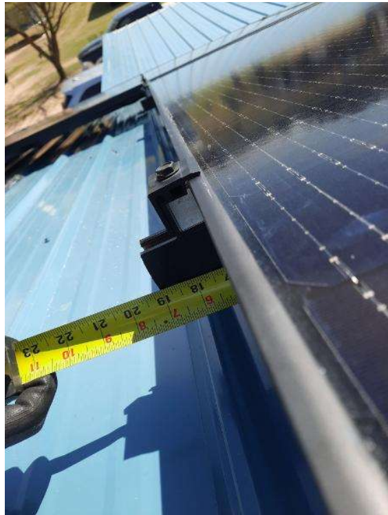
PV Arrays / Provide a photo of ALL rail cantilevers with measurements. "Cantilever" is how far the rail extends from the last mount at the edge of an array.
