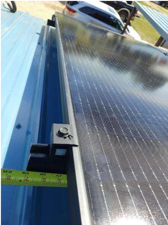
PV Arrays / Provide a photo of ALL rail cantilevers with measurements. "Cantilever" is how far the rail extends from the last mount at the edge of an array.
