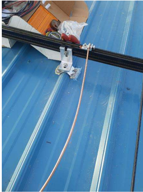
PV Arrays / Take an up close photo of EACH rail bonding lug with proper grounding wire installed.
