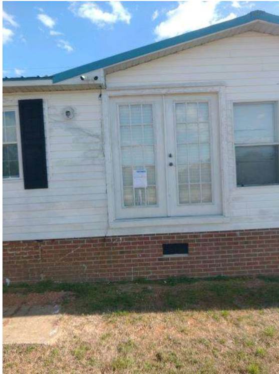
Completion / Upload a photo of location of plans left on site.
