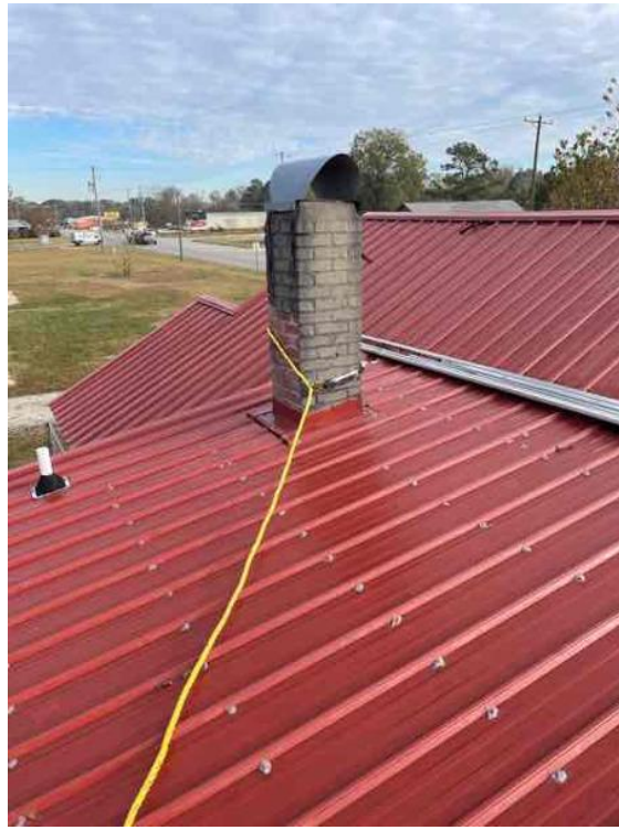
Roof / Techo / Safety Anchor Penetrations (flashed and sealed)
