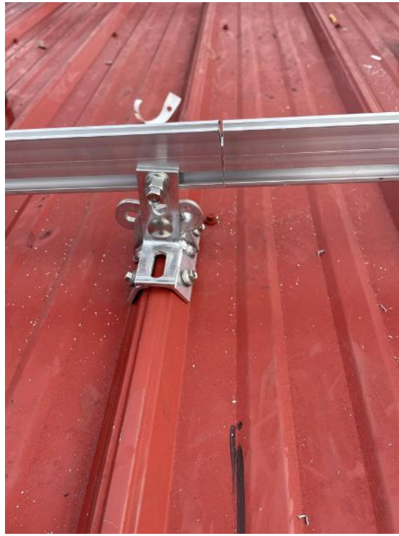
Roof / Techo / Rail Splices
