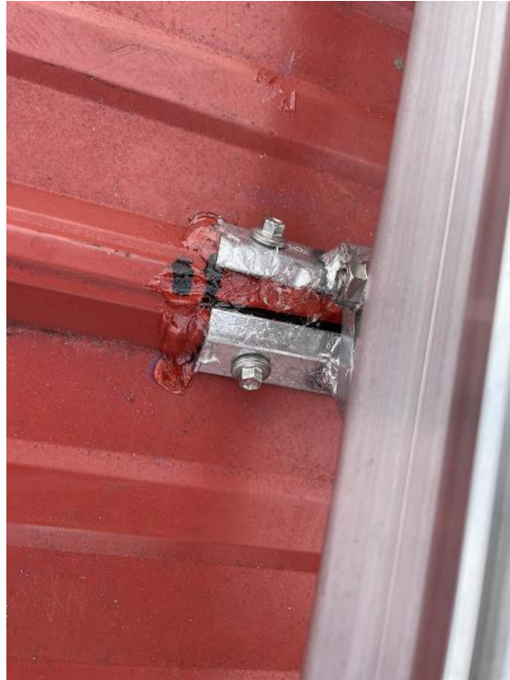
Roof / Techo / Attachment Sealant
