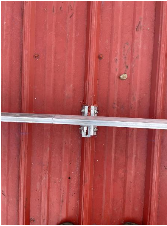
Roof / Techo / Attachment Sealant
