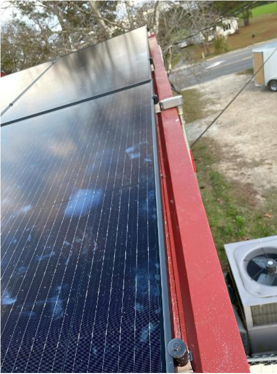
Roof / Techo / Module Clamps (Mids and Ends)
