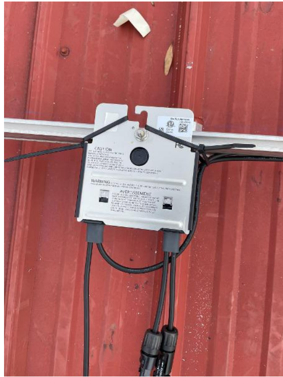
Roof / Techo / Optimizer/Microinverter Mounted
