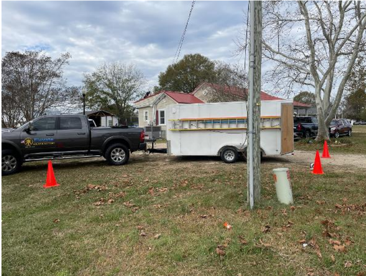
Crew & Safety / Instaladores y Seguridad / Install Vehicles w/ Safety Cones
