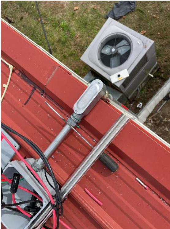
Roof / Techo / Complete Roof Conduit and Supports, with Flashing and Sealant
