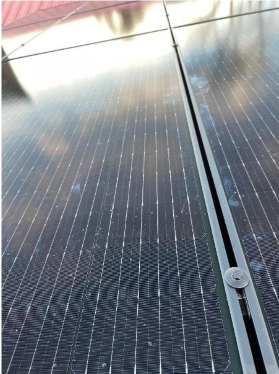
Roof / Techo / Module Clamps (Mids and Ends)
