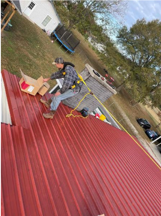
Crew & Safety / Instaladores y Seguridad / Crews Wearing Fall Protection/PPE
