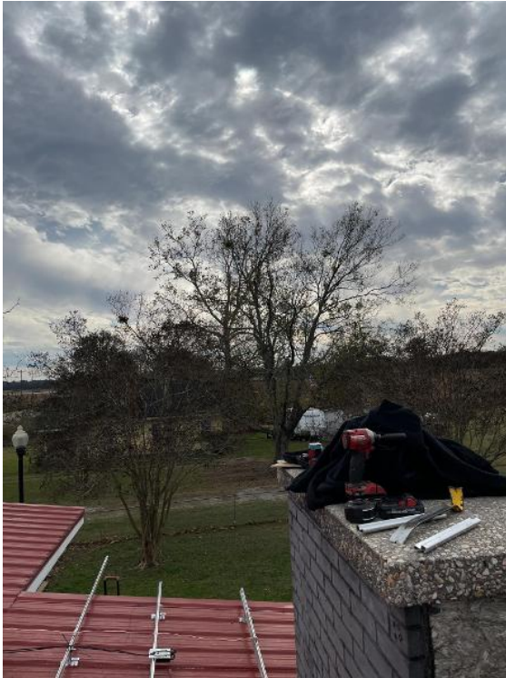
Roof / Techo / Potential Shading
