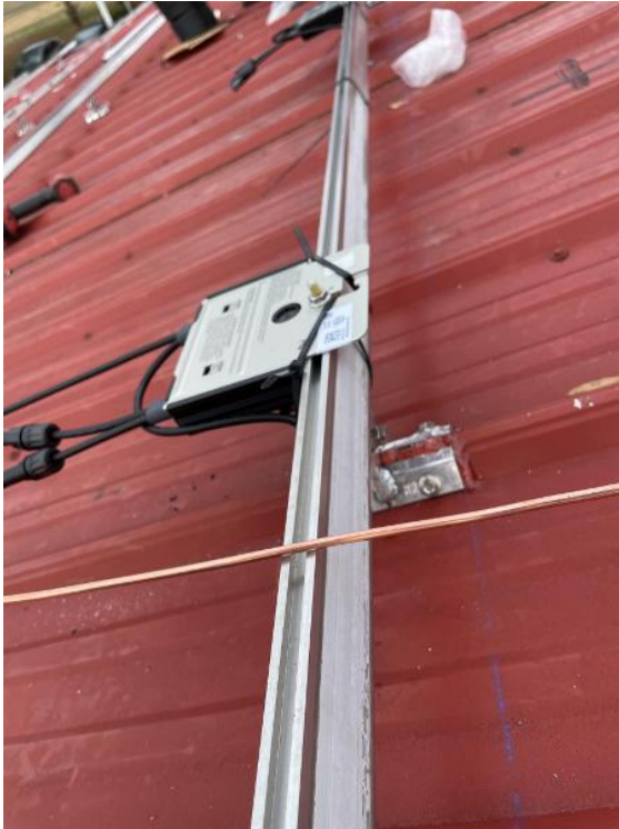
Roof / Techo / Optimizer/Microinverter Mounted
