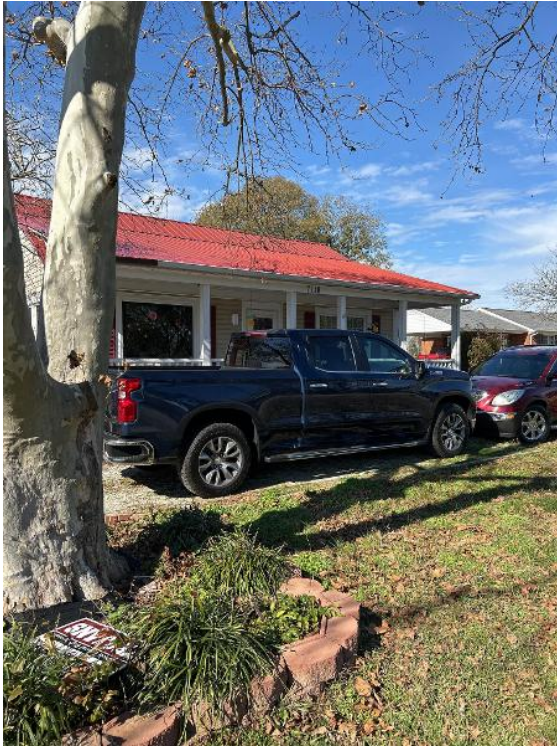
Customer Information / Informacion Del Cliente / Front of Home & Street Numbers Close Up
