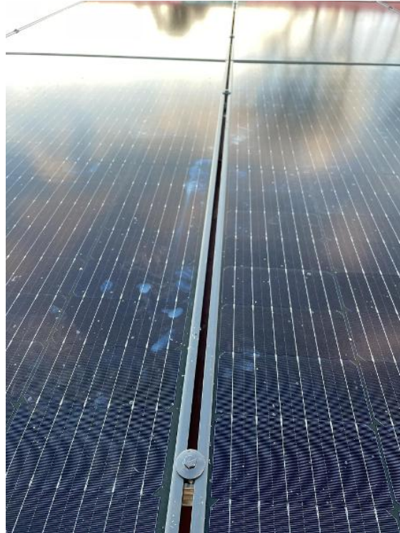
Roof / Techo / Module Clamps (Mids and Ends)
