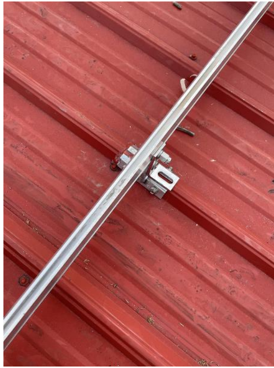
Roof / Techo / Roof Attachment (closeup and overview)
