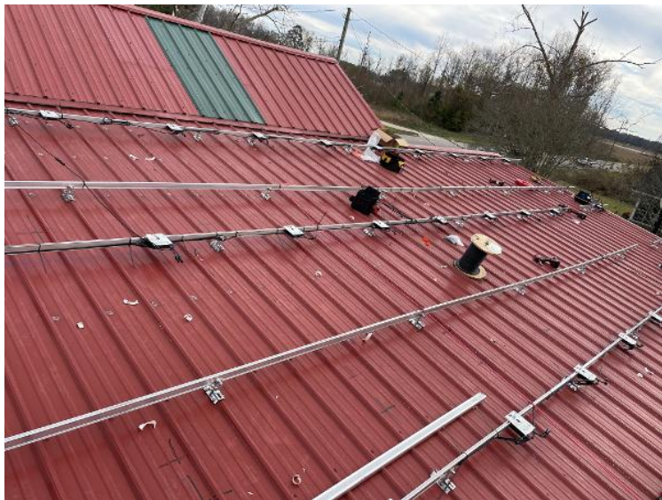
Roof / Techo / Racking and Wire Management (all arrays modules off)
