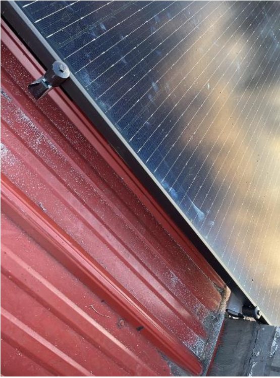
Roof / Techo / Module Clamps (Mids and Ends)
