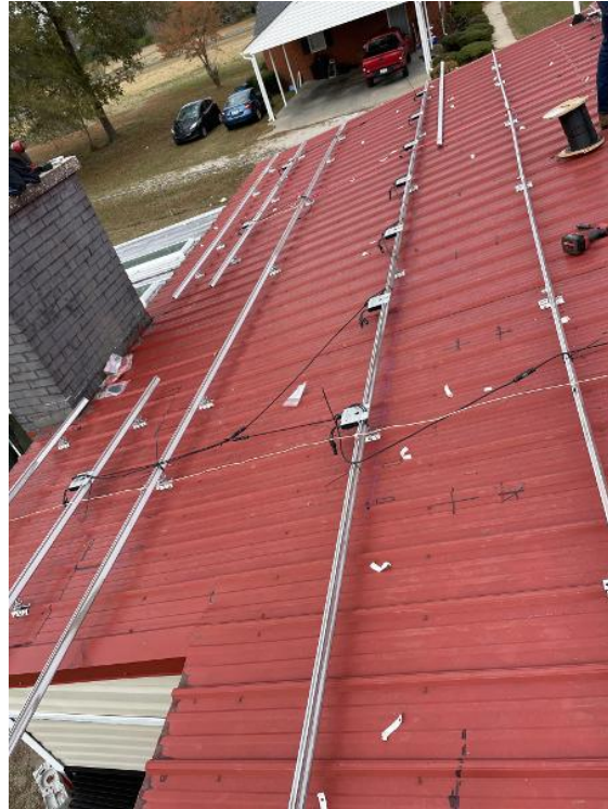
Roof / Techo / Racking and Wire Management (all arrays modules off)
