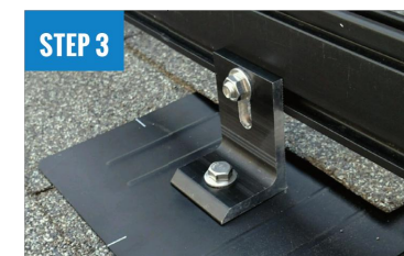
ATTACH L-FOOT TO RAIL
