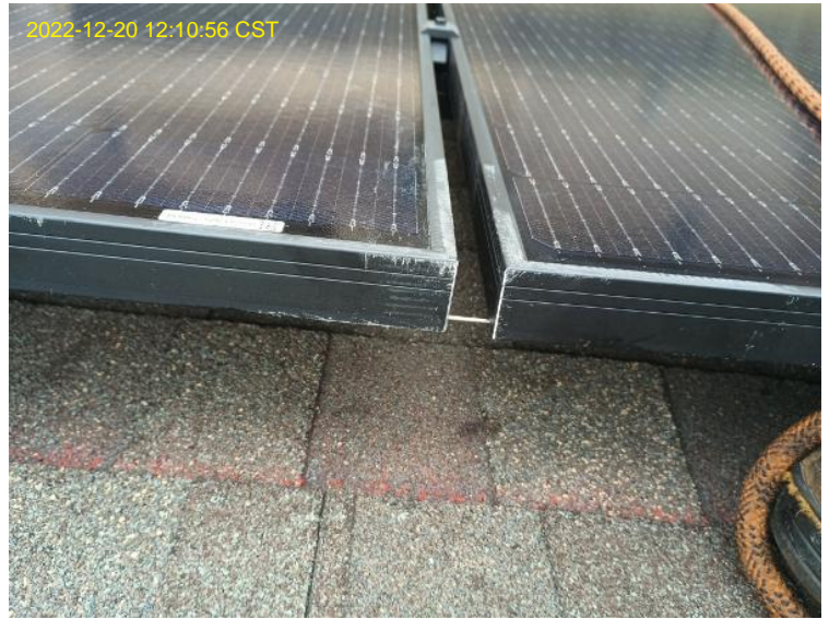
Roof/Array Work / Photo: Array Grounding Jumper(s)
