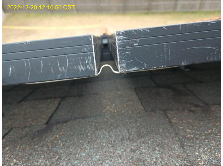
Roof/Array Work / Photo: Array Grounding Jumper(s)
