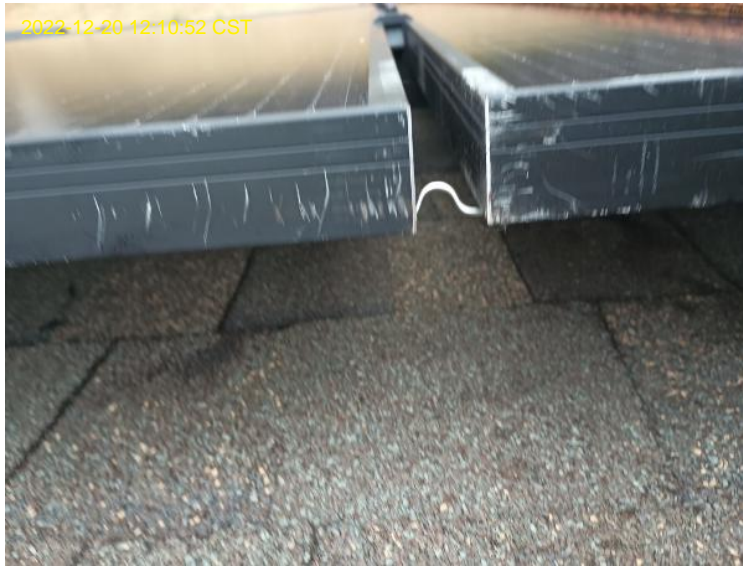
Roof/Array Work / Photo: Array Grounding Jumper(s)
