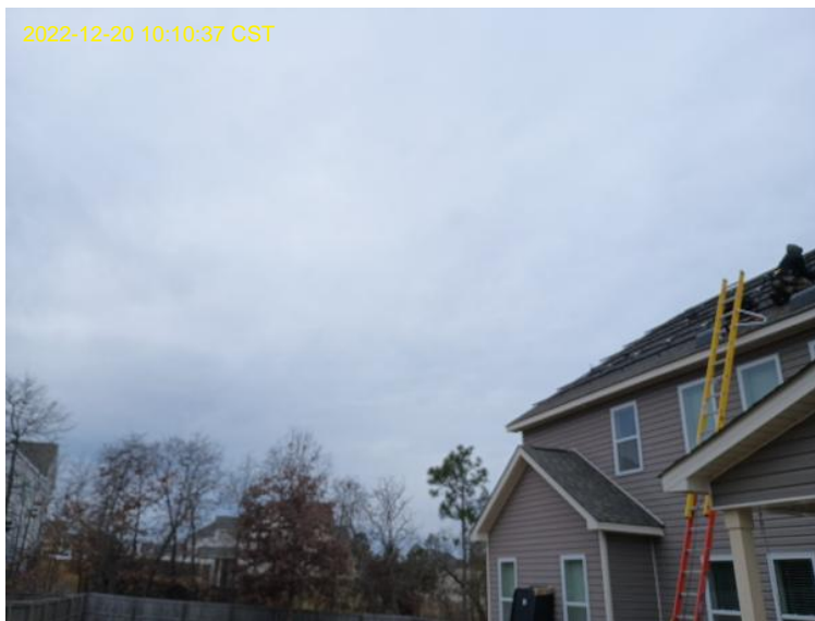
Roof/Array Work / Photo: Flashing/Roof Mount wide shot (racking)
