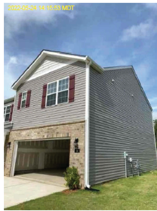
UTILITY COMPANY: Duke Energy NC
