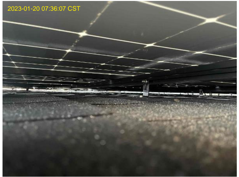
Roof/Array Work / Photo: Under Array (wire management)
