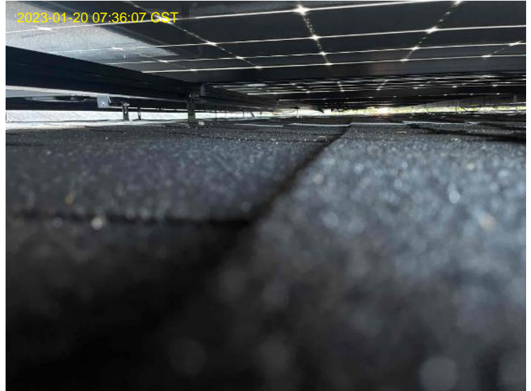
Roof/Array Work / Photo: Under Array (wire management)
