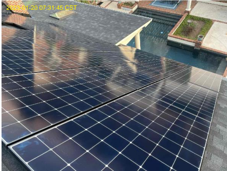
Roof/Array Work / Photo: Overall Array (s)
