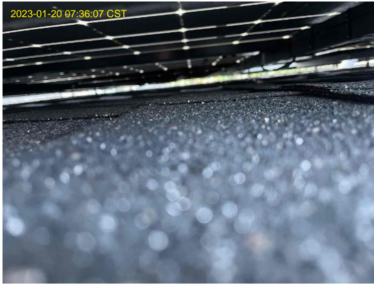
Roof/Array Work / Photo: Under Array (wire management)
