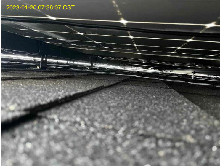
Roof/Array Work / Photo: Under Array (wire management)
