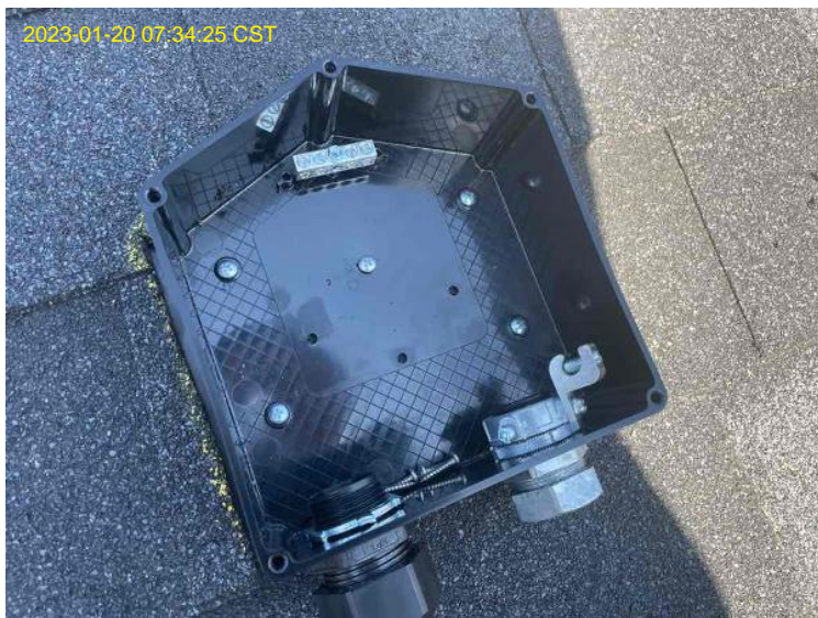
Roof/Array Work / Photo: Junction Box Wiring
