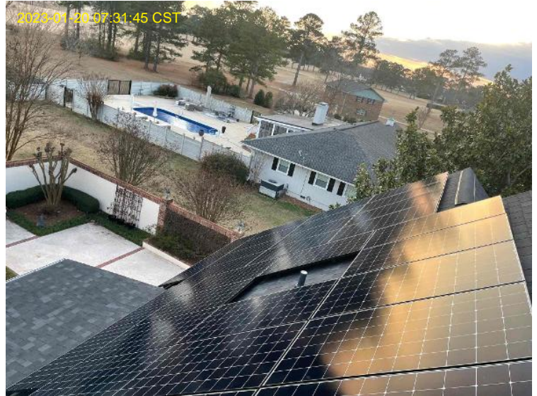
Roof/Array Work / Photo: Overall Array (s)
