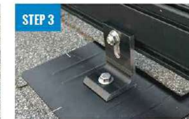
ATTACH L-FOOT TO RAIL
