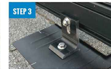
ATTACH L-FOOT TO RAIL
