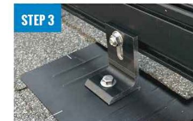
ATTACH L-FOOT TO RAIL
