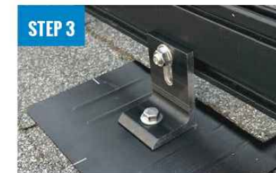
ATTACH L-FOOT TO RAIL
