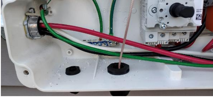
Electrical / GEC (Grounding Electrode Conductor) - main GEC (photo of the home's grounding system, MSP overview if none found)
