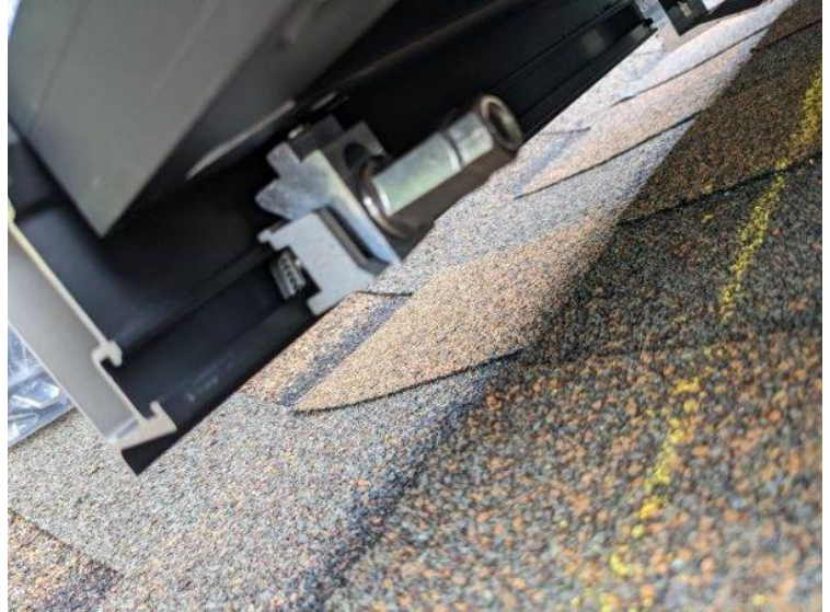
Roof / Trim Rail Grounding: 1) Take an up close photo of the trim rail bonding lug.
