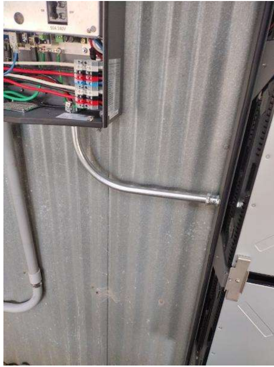
Electrical / Is there a levered battery disconnect?
