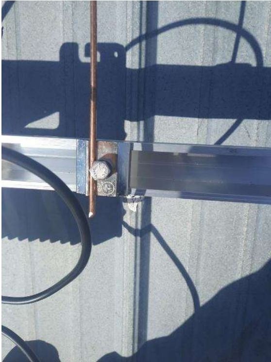
PV Arrays / Take an up close photo of EACH rail bonding lug with proper grounding wire installed.
