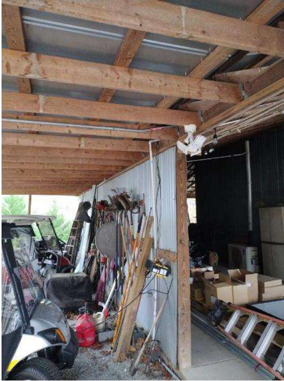
Electrical / Path To Array Roof/Attic - Conduit run, snap some shots showing the conduit is labled and secured properly.
