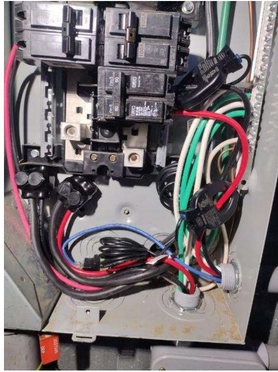
Electrical / Consumption CTs installed
