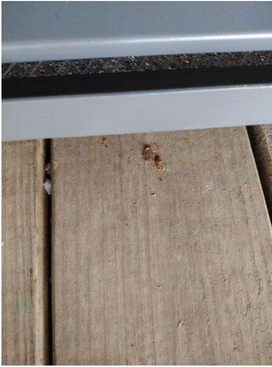
Electrical / Air intake filter installed in the cabinet
