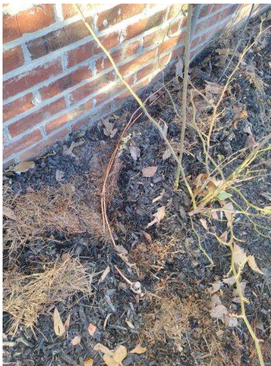
Electrical / GEC (Grounding Electrode Conductor) - Main GEC (photo of the home's grounding system)
