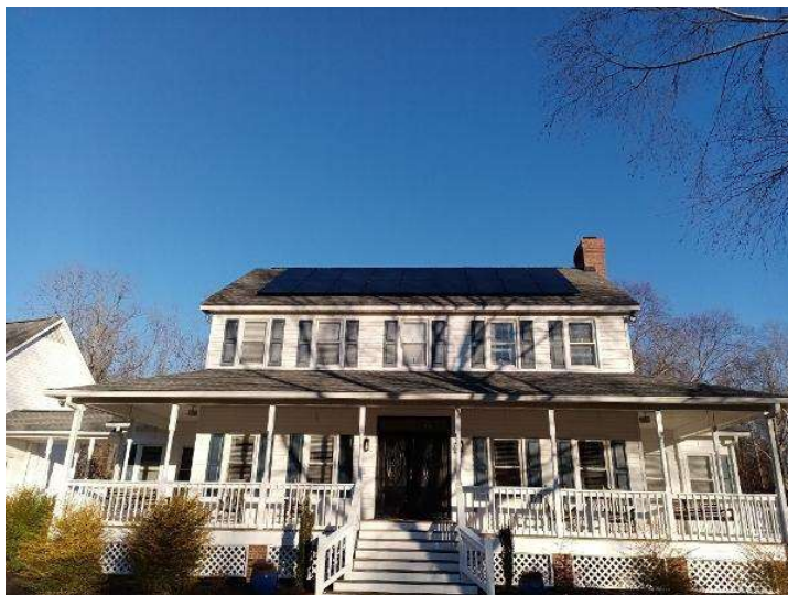
PV Arrays / Completed Array(s) showing COMPLETE overview of arrays with clean panels (No smears, handprints etc..) 3 pics per array from different angles showing each ENTIRE array.
