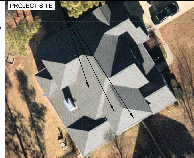
2 HOUSE PHOTO PV-1 SCALE: NTS
