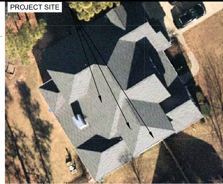
2 HOUSE PHOTO PV-1 SCALE: NTS
