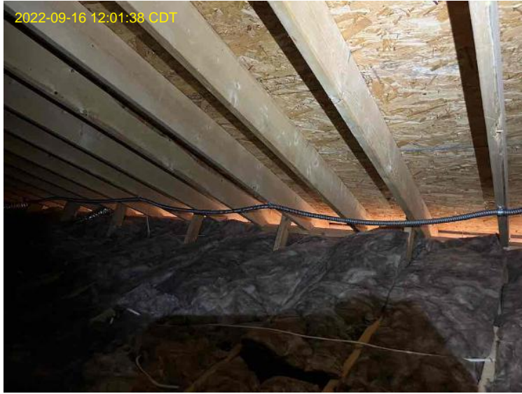
Roof/Array Work / Photo: Roof-to-Wall Transition
