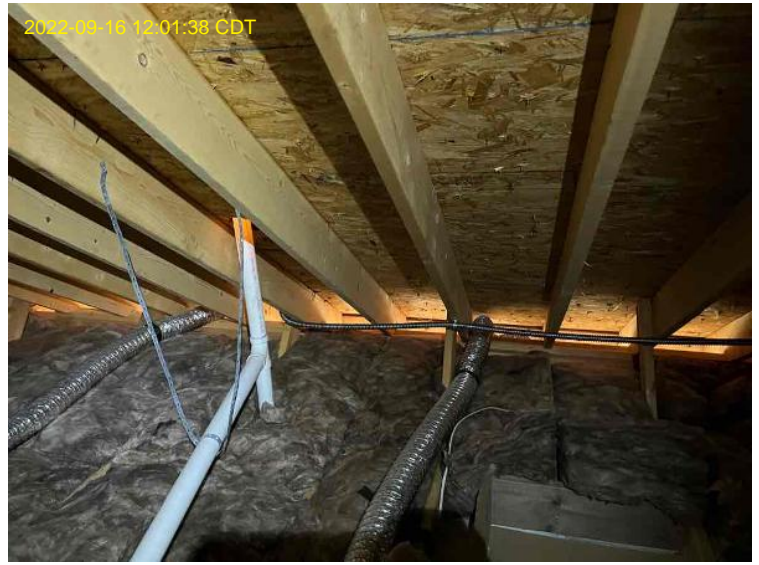
Roof/Array Work / Photo: Roof-to-Wall Transition
