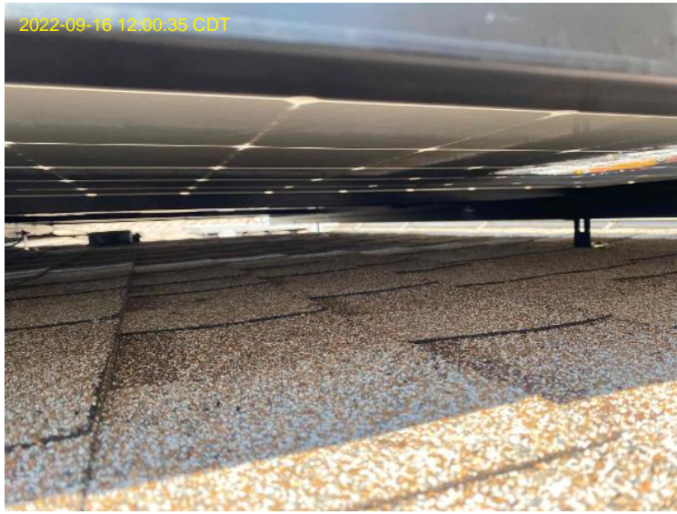
Roof/Array Work / Photo: Under Array (wire management)
