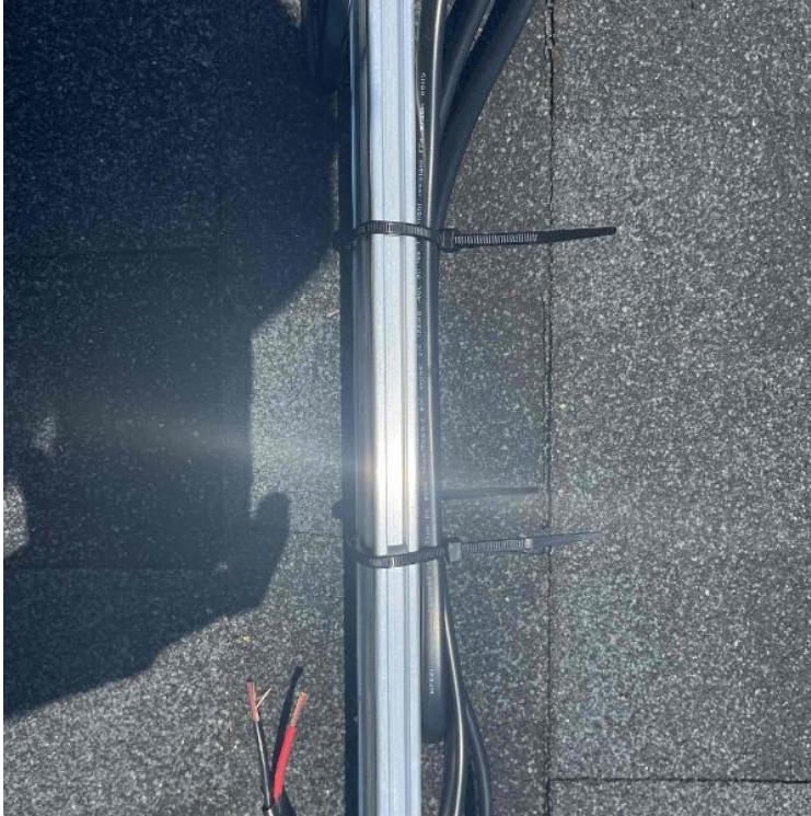
Smart Sun Energy (Super Nova Solar, LLC) Loc: 35.2355, -78.965
