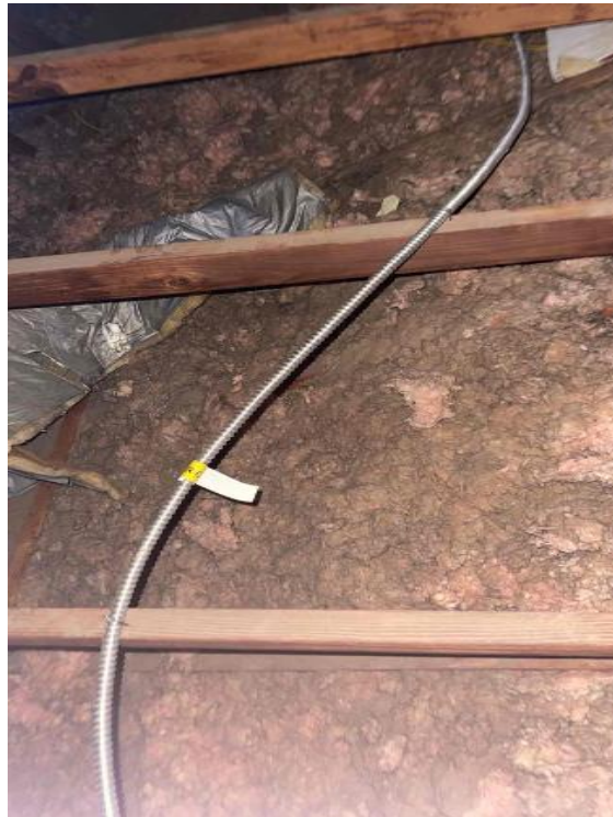
Smart Sun Energy (Super Nova Solar, LLC)
