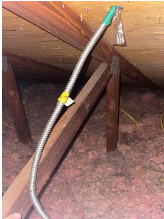
Smart Sun Energy (Super Nova Solar, LLC)
