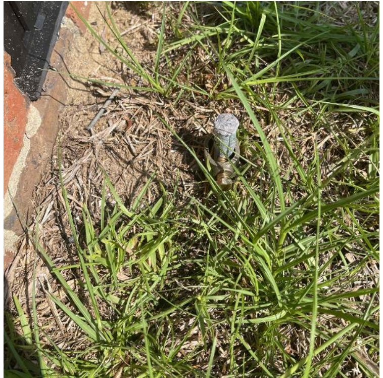
Smart Sun Energy (Super Nova Solar, LLC) Loc: 35.2355, -78.9651
