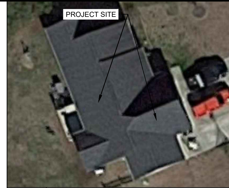
2 HOUSE PHOTO PV-1 SCALE: NTS
