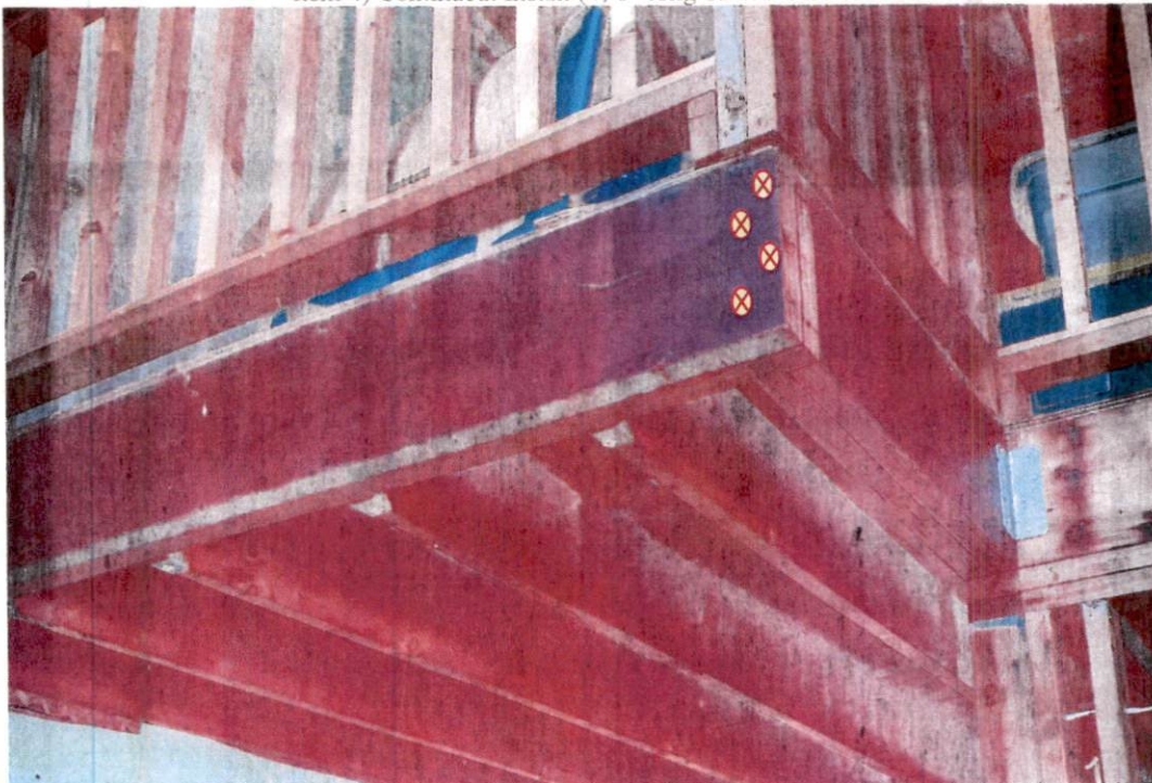
Item 5) Base Formwork Wall and Ties
