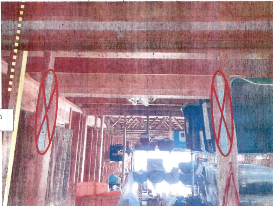
Item 4) Incorrectly installed Simpson ML28Z Connector
