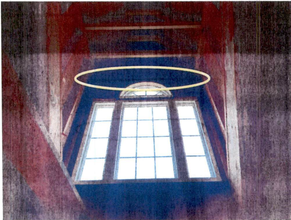
Item 3) Install Simpson LSTA12 Strap Per Plan
