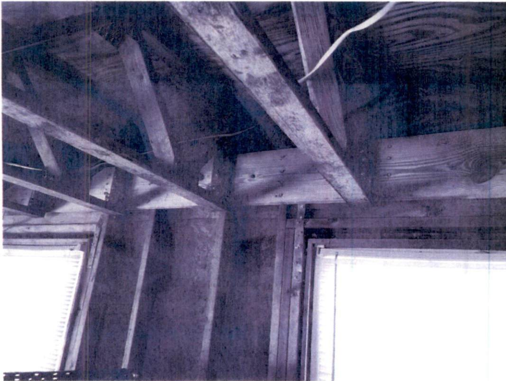
Item 6) Garage Door Studs and Blocking
