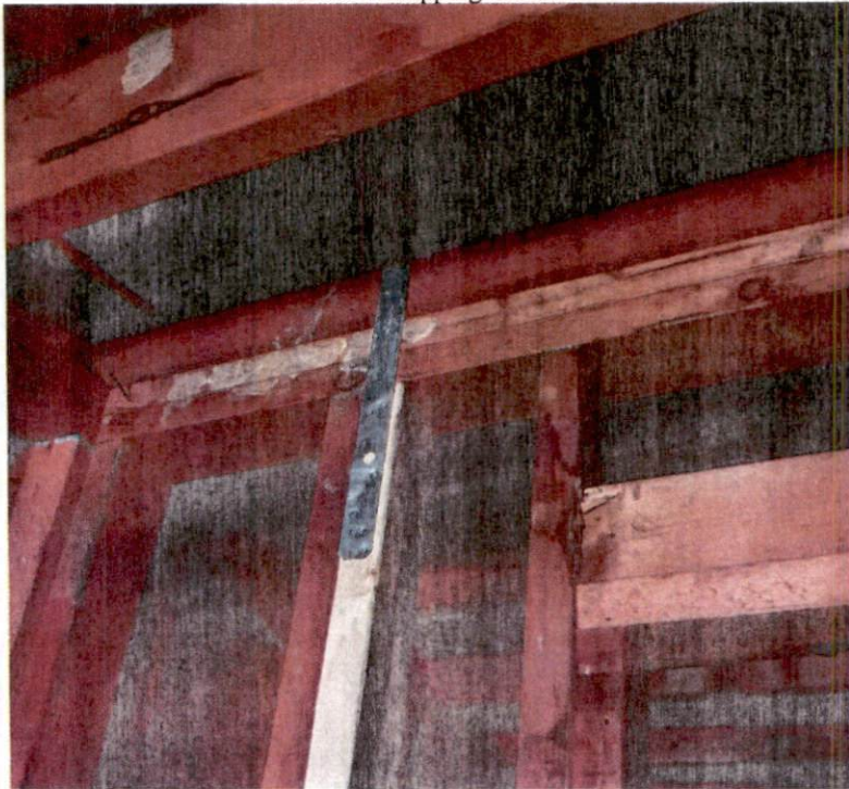
ML28Z Hanger Installed
