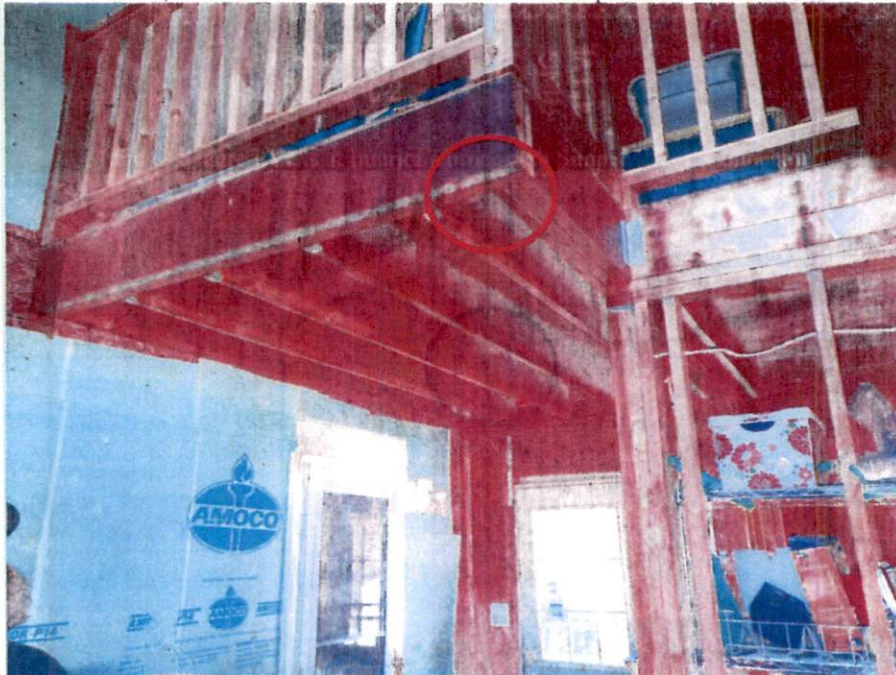
Item 6) Secure LVL's at Interior Corner with Simp. ML26Z Connector
