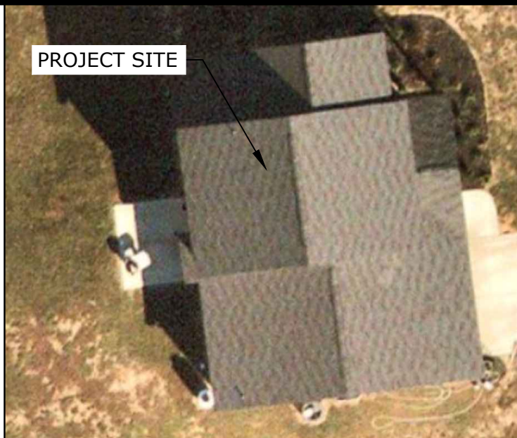
2 HOUSE PHOTO PV-1 | SCALE: NTS
