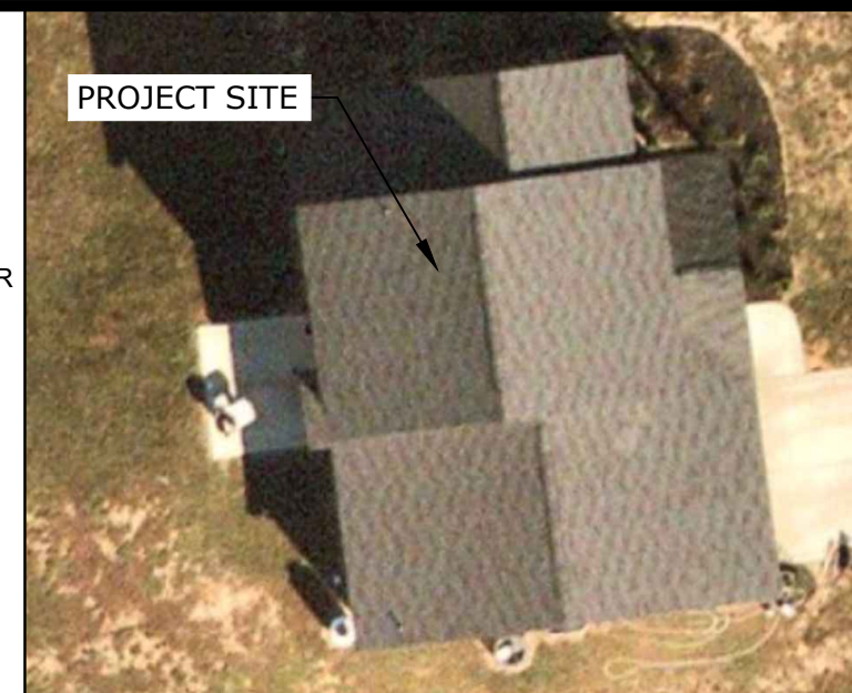
2 HOUSE PHOTO PV-1 | SCALE: NTS
