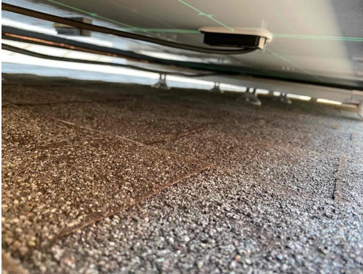
Roof / Wire Management - Quality pictures (need to show the entire array under the panel through pictures.absolutely no dangling wires)
