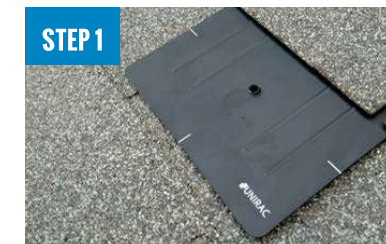
STEP 1 INSTALL FLASHKIT PRO FLASHING
