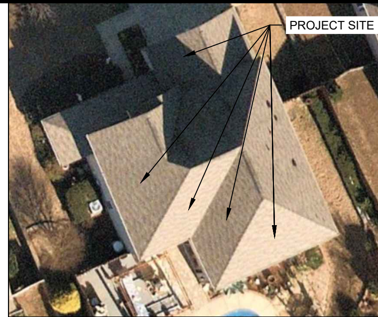
2 HOUSE PHOTO PV-1 SCALE: NTS
