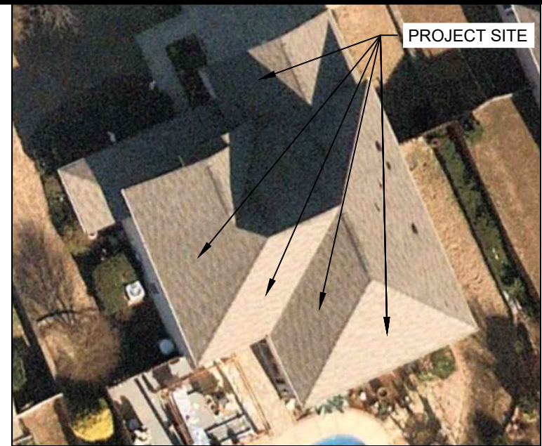
2 HOUSE PHOTO PV-1 SCALE: NTS
