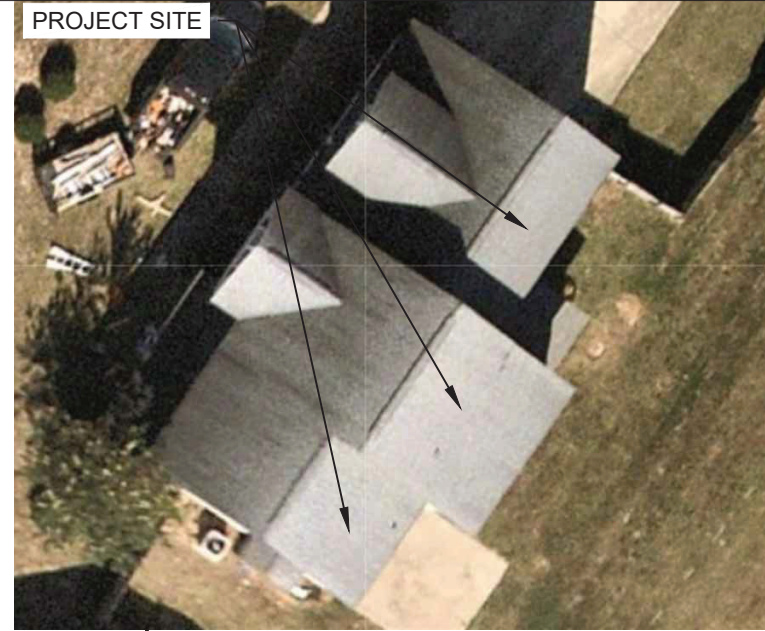
2 HOUSE PHOTO PV-1 | SCALE: NTS
