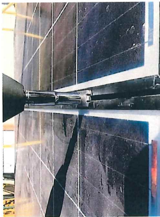
5. TIGHTEN T-BOLT SO THAT MIDCLAMP IS PERPENDICULAR TO RAIL SPLICE.
