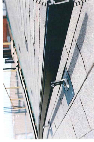
8. SEE RAIL ATTACHED TO L-FOOT.
