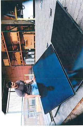
5. INSERT SECOND MODULE INTO PLACE.
