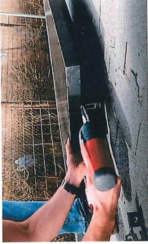
3. WHILE HOLDING MODULE IN POSITION AND WITH FLANGE IN FULL CONTACT WITH RAIL, USE DRILL TO ROTATE END CLAMP BOLT UNTIL CLAMP ENGAGES WITH FLANGE TO PROVIDE CLAMP FORCE.
