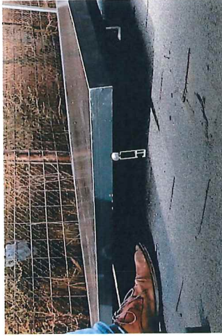
4. SEE MODULE ENGAGED BY ENDCLAMP.
