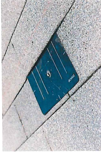
2. INSERT THE FLASHING SO THE TOP PART IS UNDER THE NEXT ROW OF SHINGLES AND THE HOLE LINES UP WITH THE PILOT HOLE.
