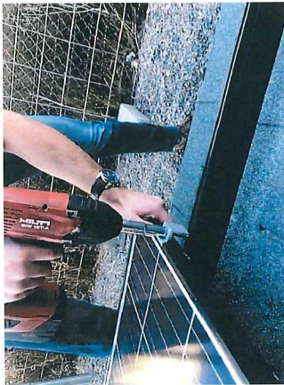
2. ENGAGE MODULE FRAME WITH ENDCLAMPS. TIGHTEN T-BOLT WITH DRILL.
