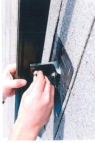
6. HAND TIGHTEN NUT UNTIL RAIL ALIGNMENT IS COMPLETE. VERIFY THAT POSITION INDICATOR ON BOLT IS VERTICAL (PER PERMITS II, AB, TO, PART 1).
