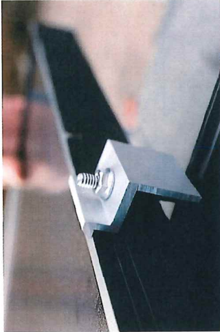
3. SEE MODULE ENGAGED BY ENDCLAMP.
