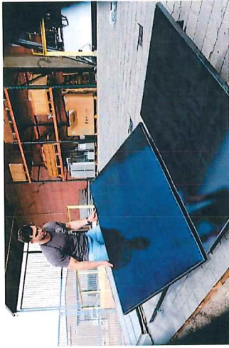
5. INSERT SECOND MODULE INTO PLACE.
