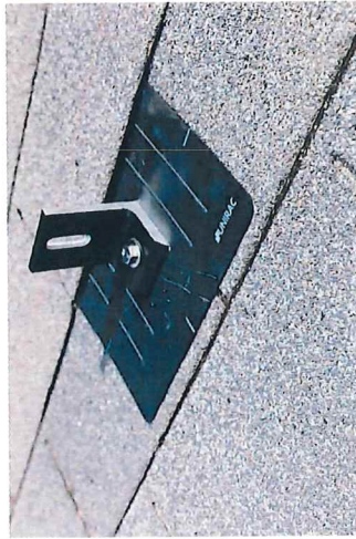
4. INSERT THE LAG BOLT THROUGH THE L-FOOT IN THE ORDER SHOWN IN THE IMAGE. VERIFY PROPER ORIENTATION BEFORE TIGHTENING LAG BOLTS.
