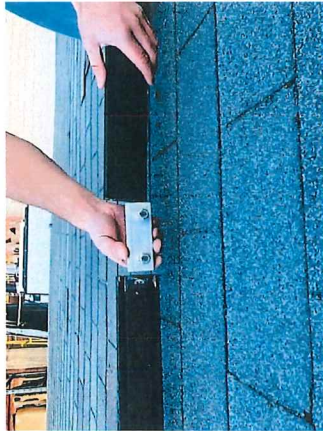
1. SLIDE T-FEATURE ON SPlice INTO THE T-SLOT ON EACH RAIL, CENTERING THE SPlice BETWEEN THE TWO RAILS.
