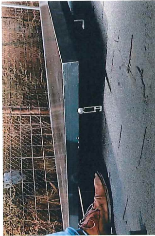
4. SEE MODULE ENGAGED BY ENDCLAMP.
