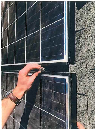
4. INSERT 1/4" T-BOLT INTO RAIL.
