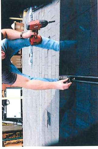
6. INSERT 1/4" T-BOLT INTO TOP SLOT OF RAIL. ENSURE BOLT IS PERPENDICULAR TO RAIL.
