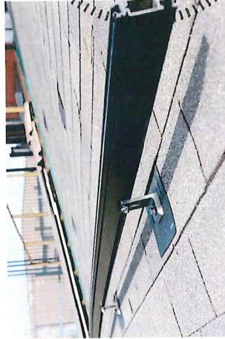
8. SEE RAIL ATTACHED TO L-FOOT.
