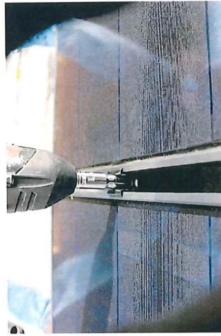
7. MODULES MUST BE TIGHT AGAINST CLAMPS WITH NO GAPS. TIGHTEN NUT.
