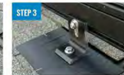
ATTACH L-FOOT TO RAIL
