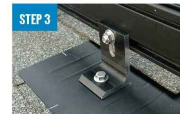
ATTACH L-FOOT TO RAIL
