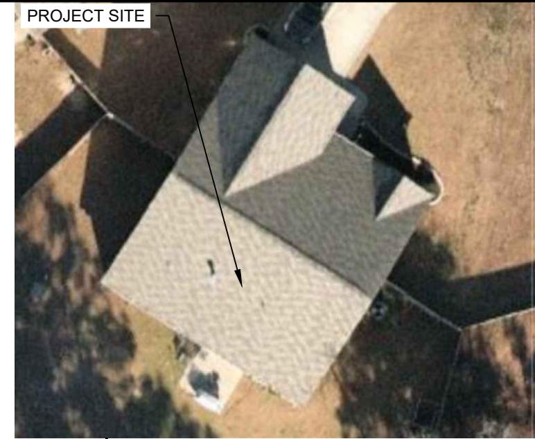
2 | HOUSE PHOTO PV-1 | SCALE: NTS
