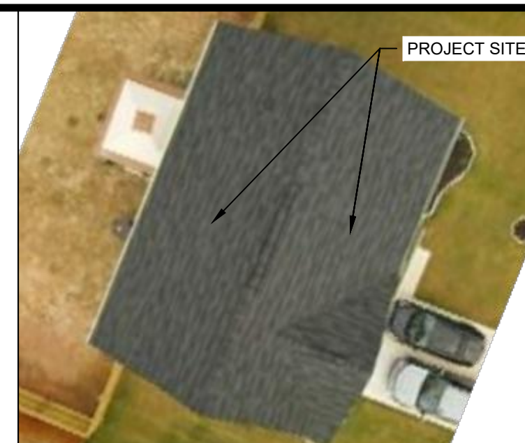
2 HOUSE PHOTO PV-1 SCALE: NTS
