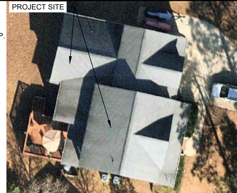
2 HOUSE PHOTO PV-1 SCALE: NTS
