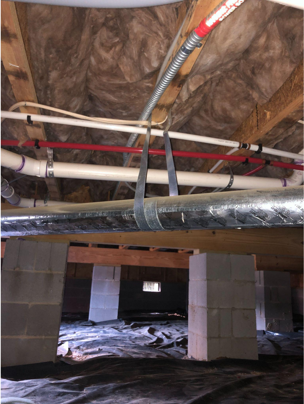
Hale, Rick, 20 Dot CourtFuquay-Varina, NC 27526- PV Inspection Pictures
