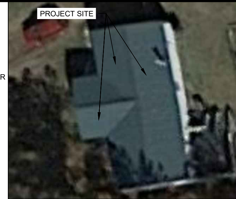
2 HOUSE PHOTO PV-1 | SCALE: NTS
