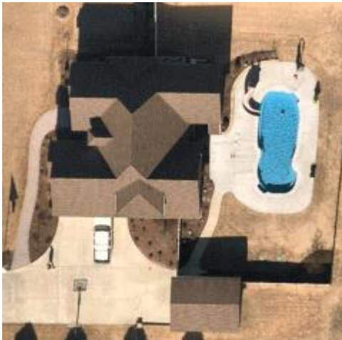
TOP VIEW OF BUILDING
