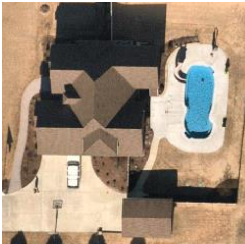
TOP VIEW OF BUILDING
