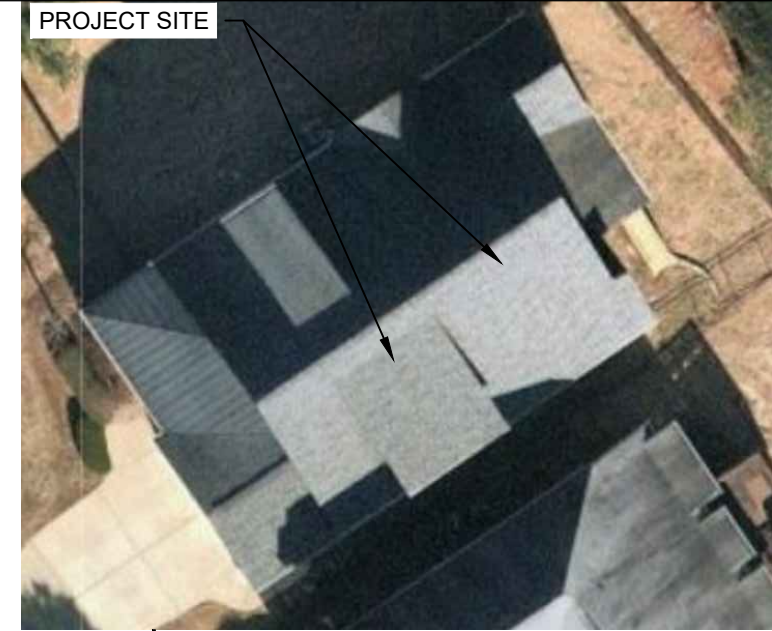
2 HOUSE PHOTO PV-1 SCALE: NTS
