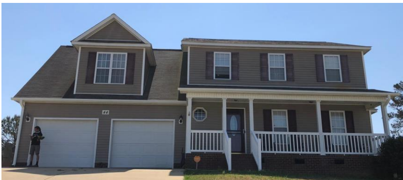
FRONT VIEW OF BUILDING
