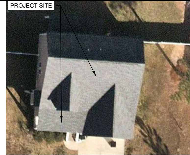
2 | HOUSE PHOTO PV-1 | SCALE: NTS
