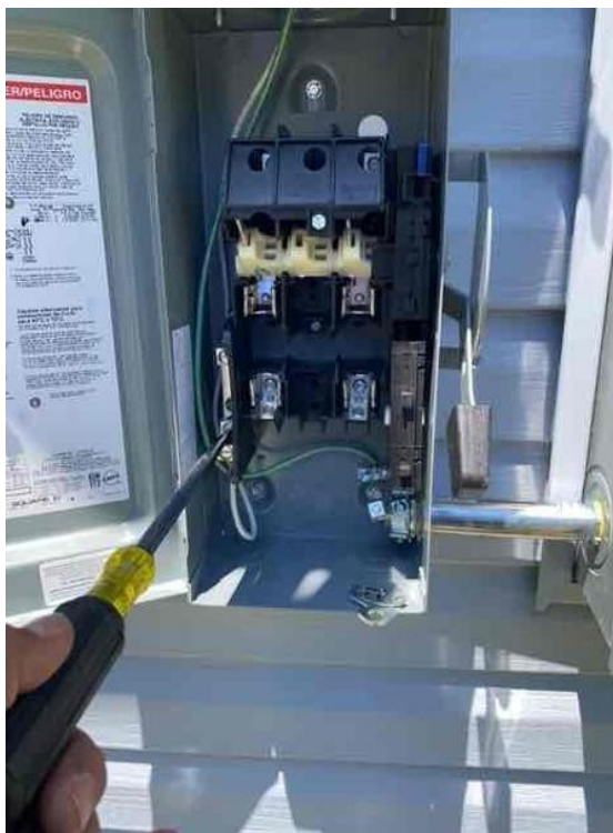
TX Dallas Crew 1
