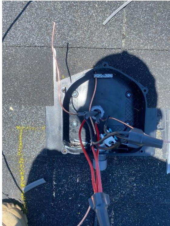
TX Dallas Crew 1 Loc: 35.5326, -78.8541
