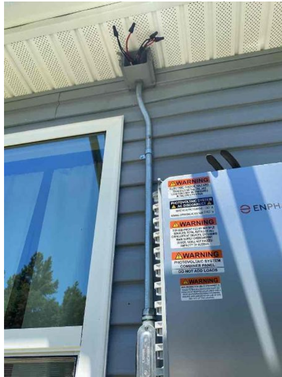
TX Dallas Crew 1
