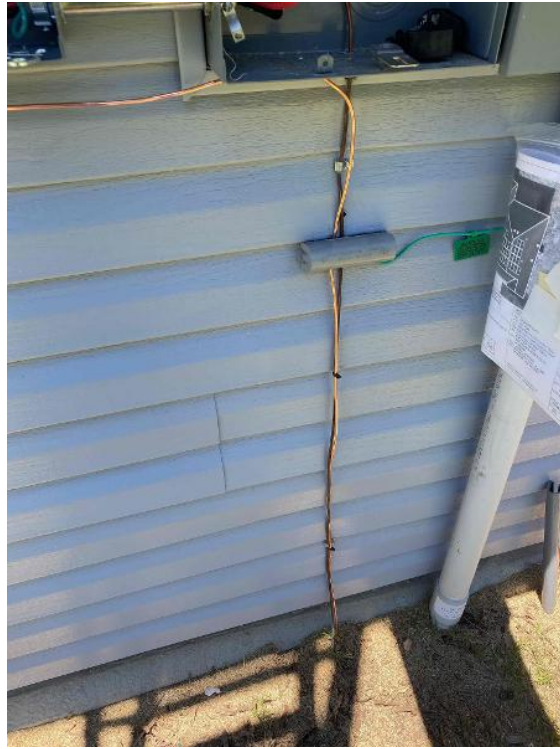
TX Dallas Crew 1
