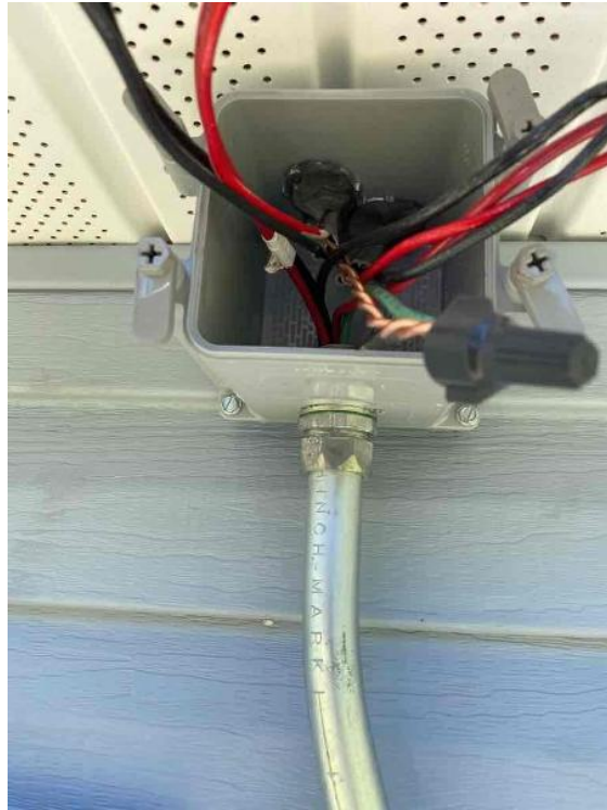
TX Dallas Crew 1
