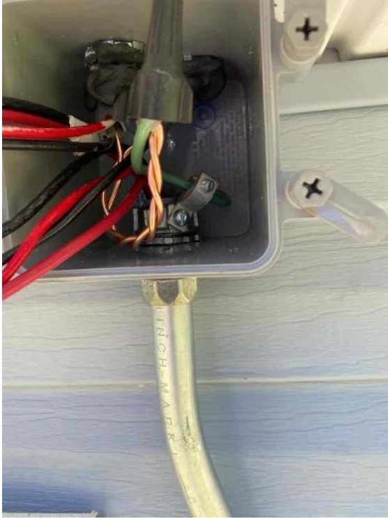
TX Dallas Crew 1
