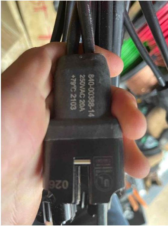
TX Dallas Crew 1
