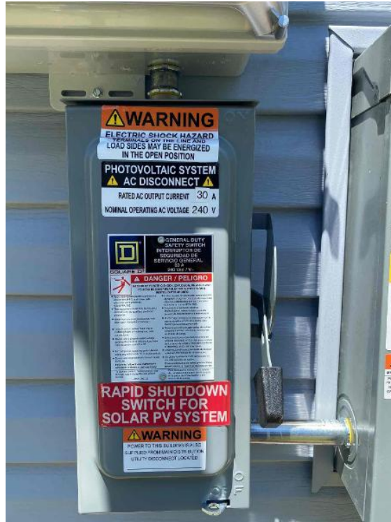
TX Dallas Crew 1
