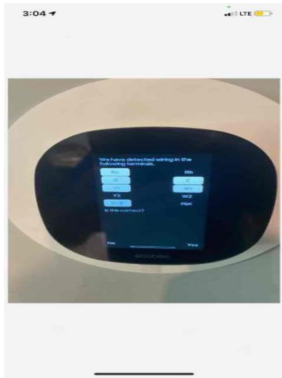
TX Dallas Crew 1
