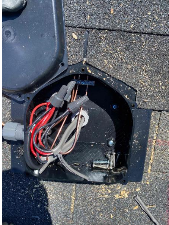
TX Dallas Crew 1 Loc: 35.5327, -78.8541
