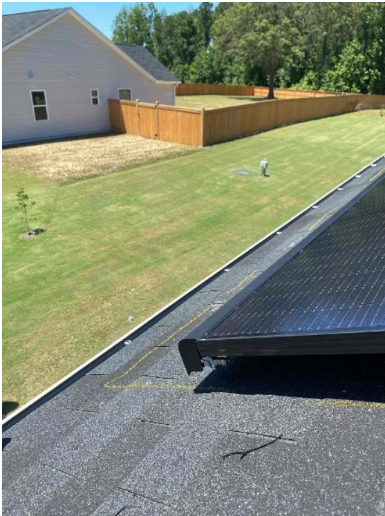
TX Dallas Crew 1 Loc: 35.5326, -78.8541
