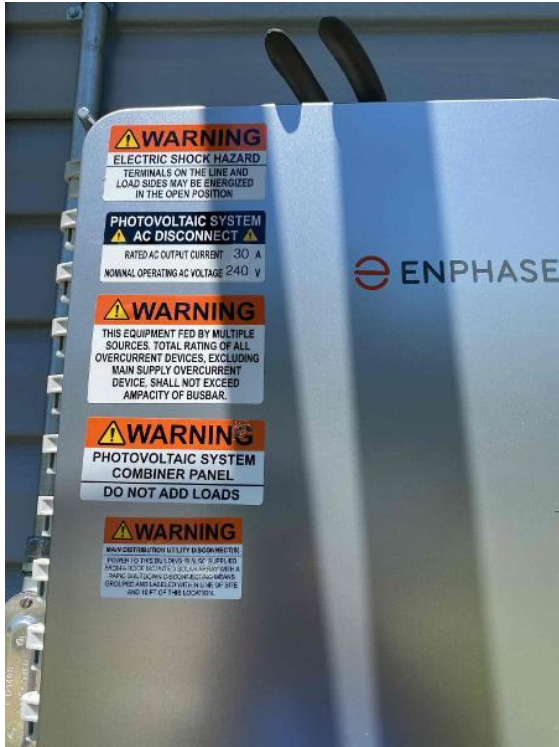
TX Dallas Crew 1
