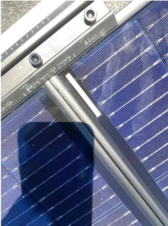
TX Dallas Crew 1 Loc: 35.5327, -78.8541
