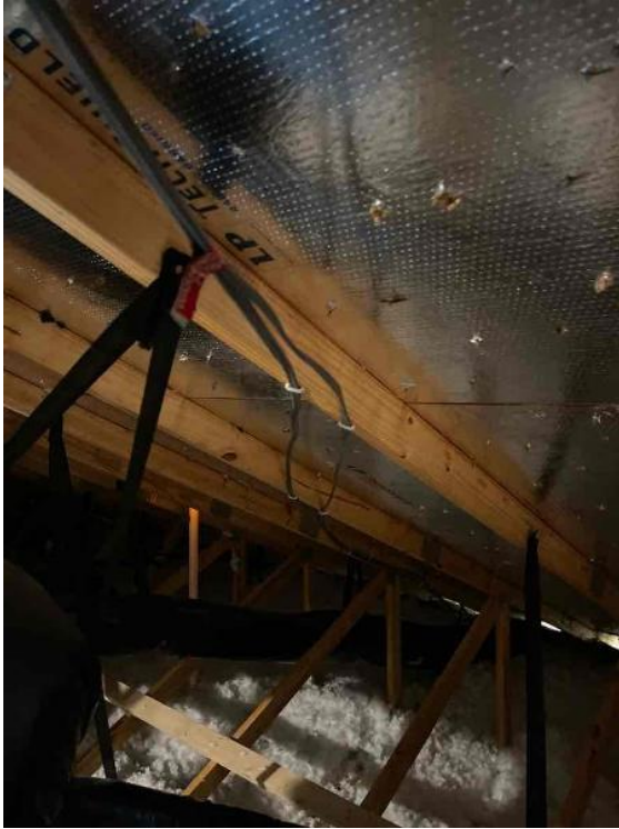
TX Dallas Crew 1 Loc: 35.5326, -78.8541
