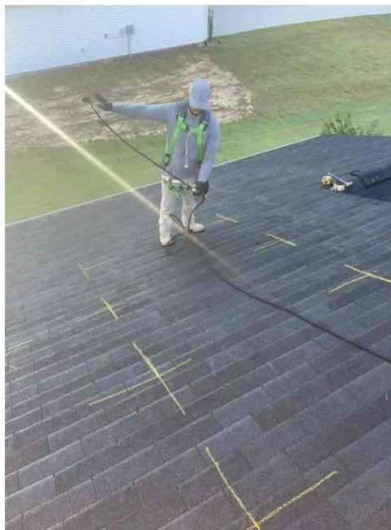
TX Dallas Crew 1 Loc: 35.5326, -78.854
