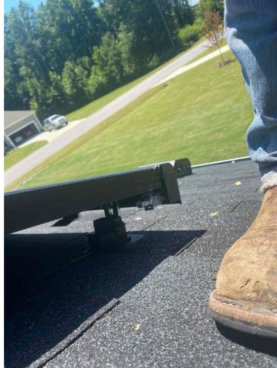
TX Dallas Crew 1 Loc: 35.5327, -78.8541
