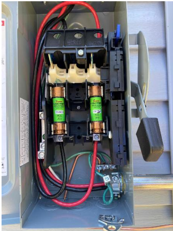
TX Dallas Crew 1
