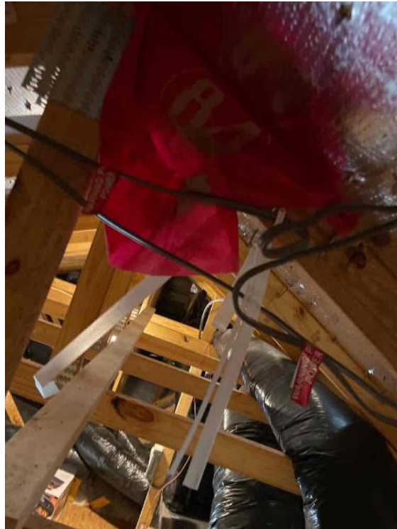
TX Dallas Crew 1 Loc: 35.5326, -78.8541
