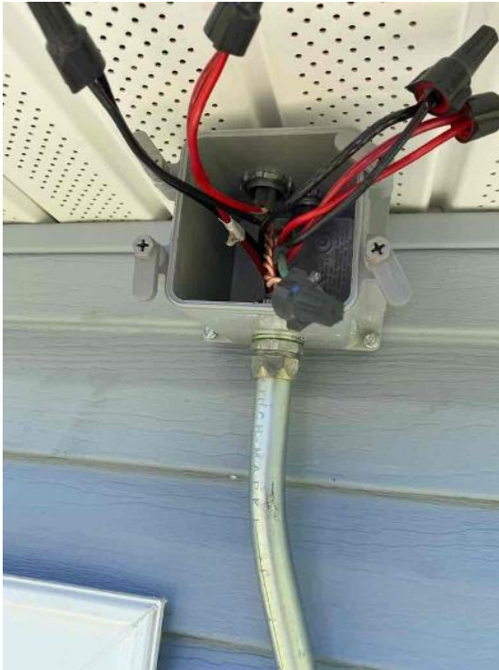
TX Dallas Crew 1
