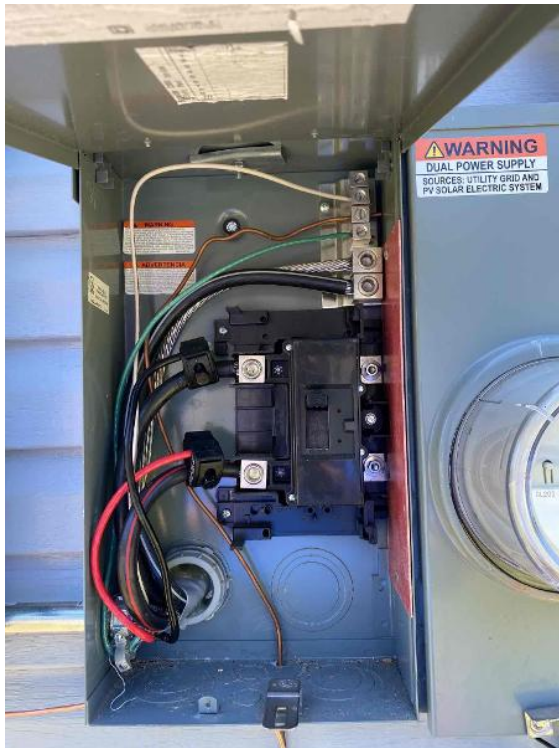
TX Dallas Crew 1
