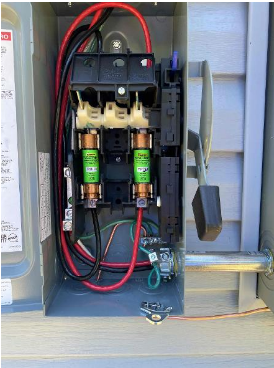
TX Dallas Crew 1
