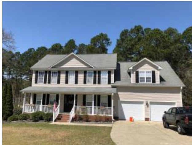
FRONT VIEW OF BUILDING
