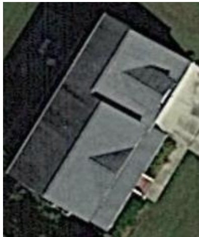
TOP VIEW OF BUILDING
