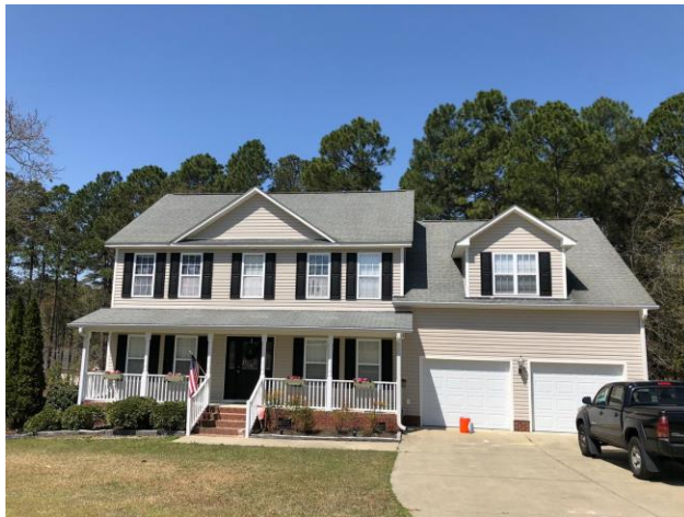
FRONT VIEW OF BUILDING
