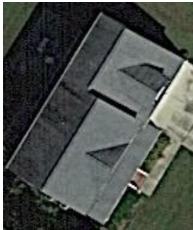
TOP VIEW OF BUILDING
